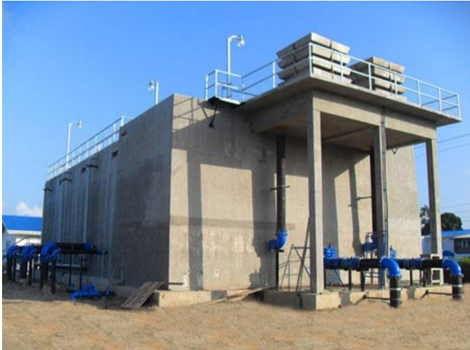
Central Ruimveldt Treatment Plant
