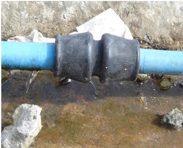
personnel to reduce water losses.
