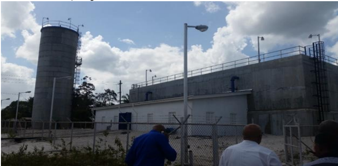
Wisroc Treatment Plant/Storage Tank
