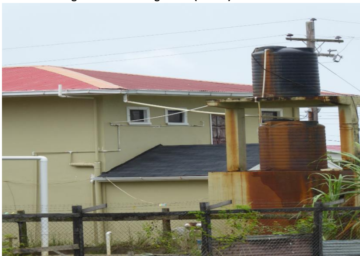
Water loss - faulty connection (above) An overflowing customer storage tank (below)
