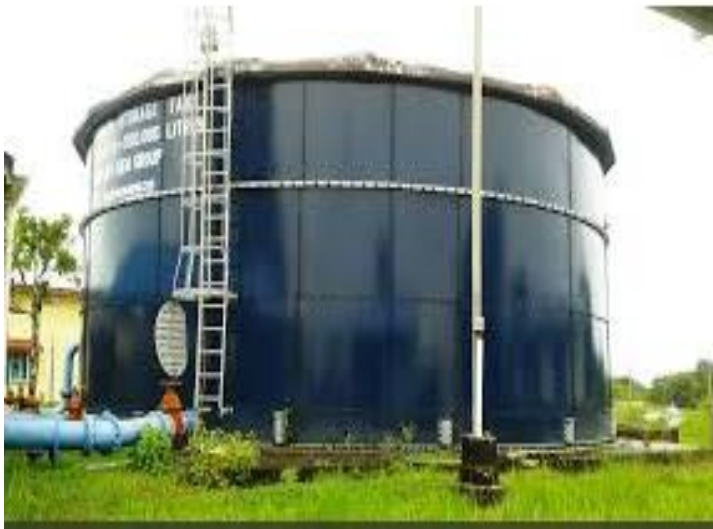
A storage Tank at Bartica
